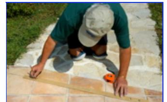
4. Remove the GATE TEMPLATE and set it aside. Then, from the centre of the outer hole measure 57mm or use the FENCE TEMPLATE, which will give you the centre of your first hole for the fencing. See Diagram 2 - Using the Fence Template
