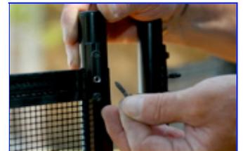
Connect the Hooks and Eyes as you go, twisting the poles if required, to create tension in the fence panel and making sure that the metal edging strip and screws are facing outwards.
